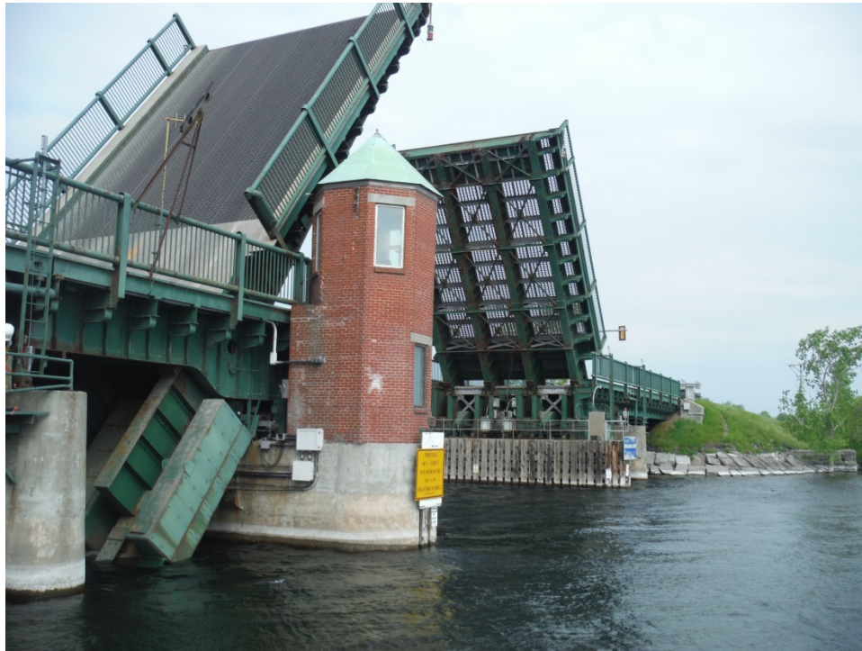
Photo showing the drawbridge back spans in the water
